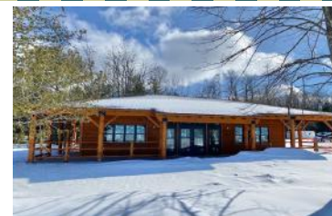
ONAWAY STATE PARK PAVILLION
